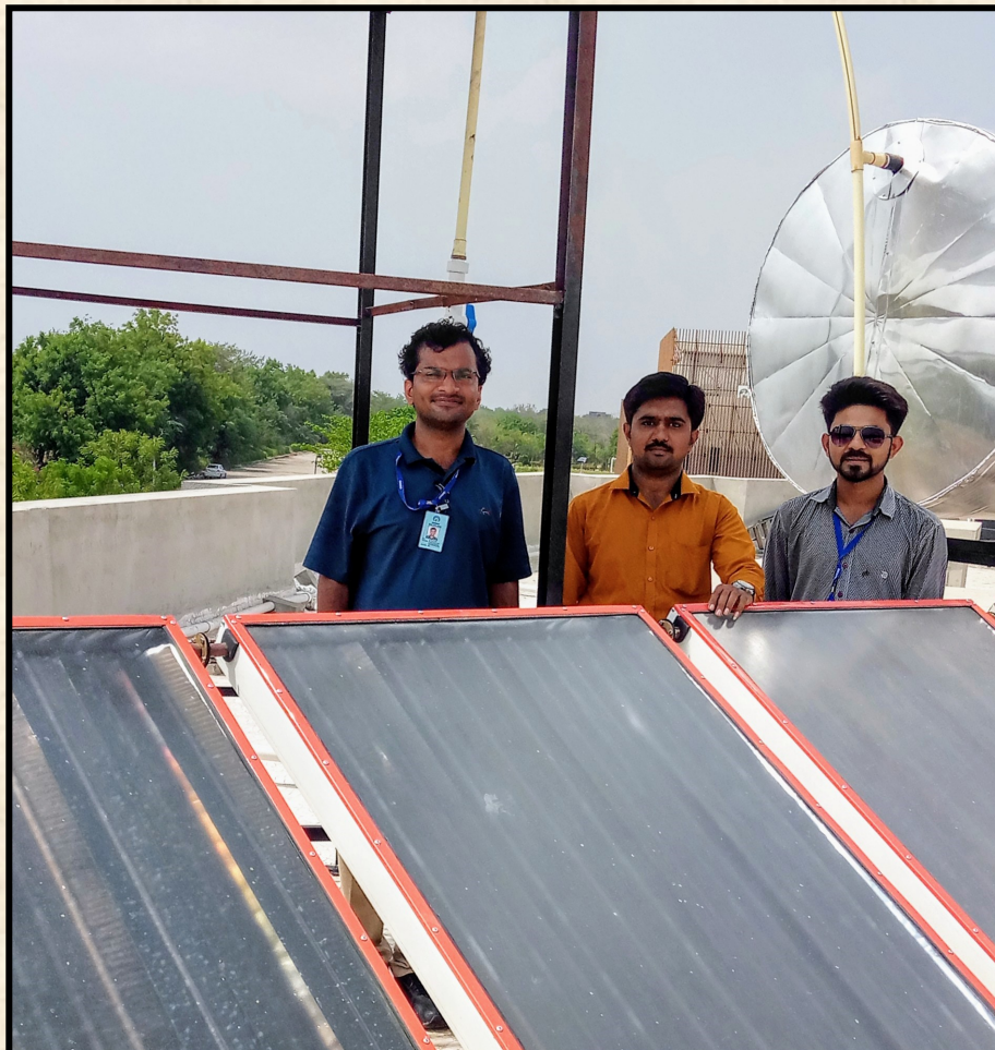
Performance testing of Solar water heating systems installed at the terrace of GNLU
